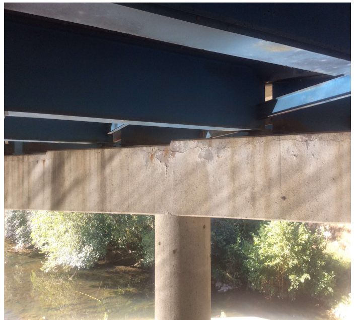
PHOTO 2 Description Bent 3 cap back . Horizontal crack up to 0.035 wide with rust stains. in the cap under beams 2,3 & 4
