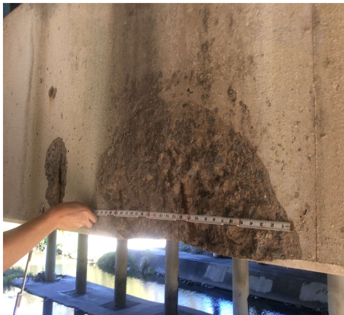
PHOTO 3 Description Bent 4 cap ahead between column 2 & 3 spalls with exposed rebar.
