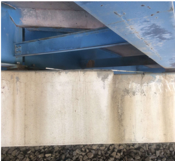
PHOTO 1 Description Bent 2 cap ahead under beams 6 & 7. The cap has a horizontal crack 13 foot long and up to 0.025" wide.
